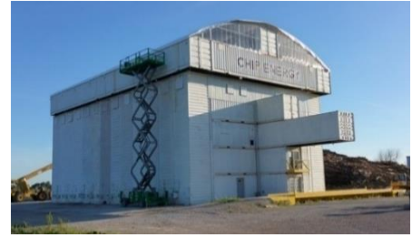
Figure 3. Chip Energy Biomass Conversion Facility.
